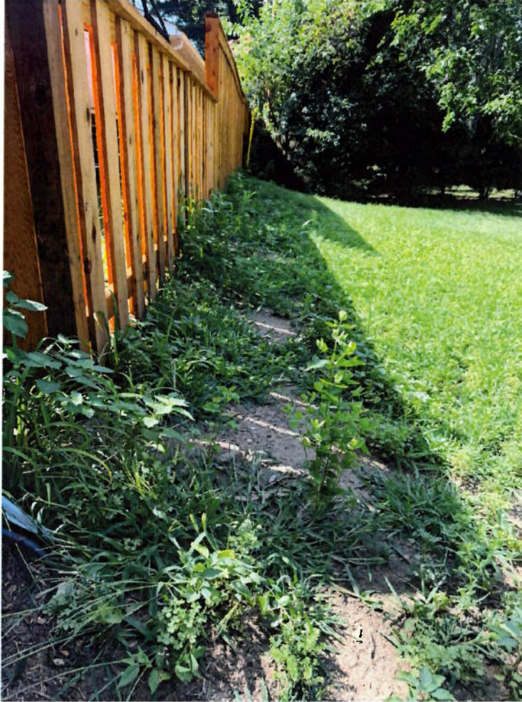
Photograph 3: 4-foot-section of fence at rear lot line. Neighbors side.
