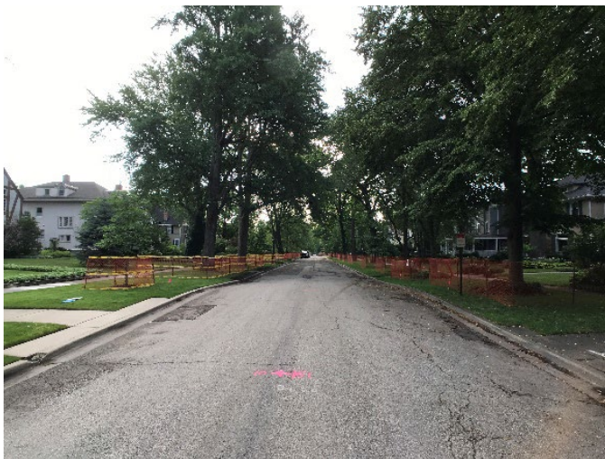
Existing Asphalt Overlay
