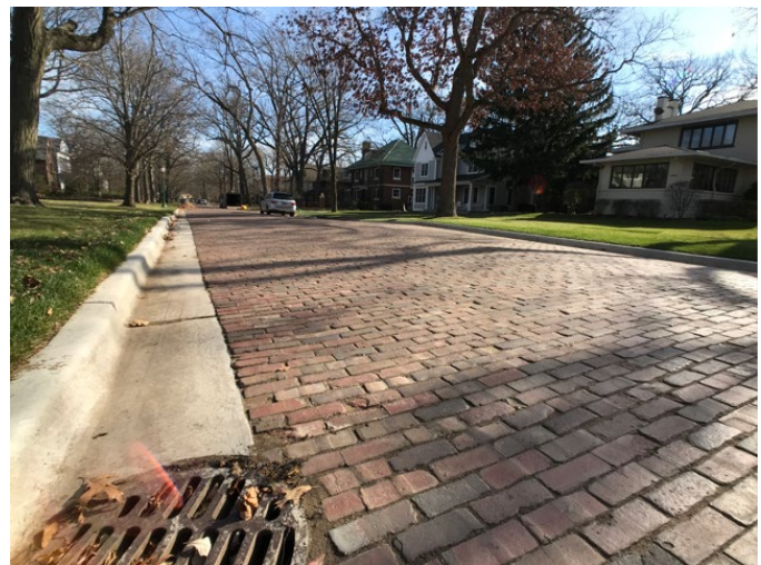
Brick Paver Reconstruction
