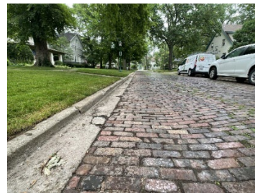
Edge After Repair
